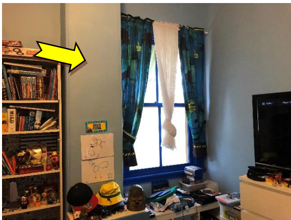
Photo 5. Exterior, boys room, walls – suspected lead-containing blue upper paint systems.
